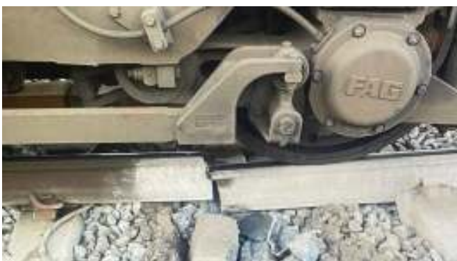
Rail break at Iver (Network Rail)
